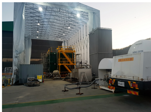
Figure 4. Pressure test in cold condition.
