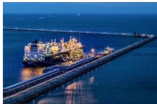
Pipe-to-LNG switch Flexibility, security of supply and reduced dependency
