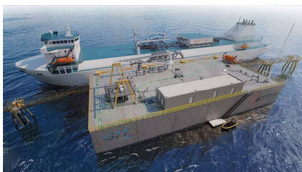
Figure 1. Acciona gravity-based structure (GBS) LNG storage concept.
