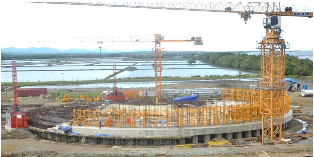
Base slab and piles
