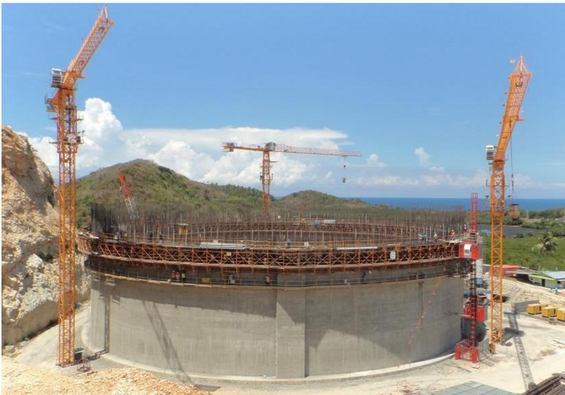
During wall pouring
