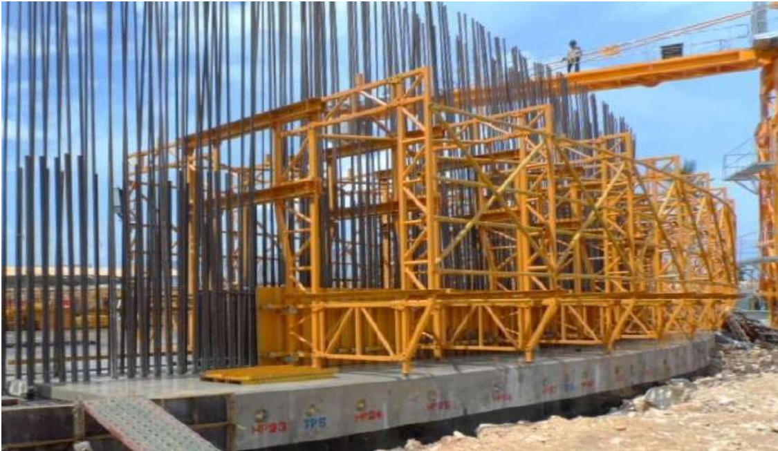
Base slab and formwork
