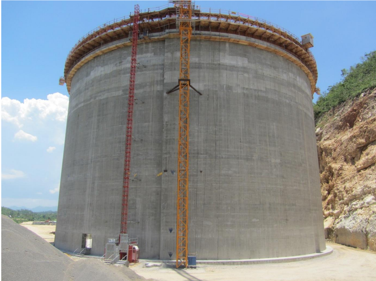
After walls completion
