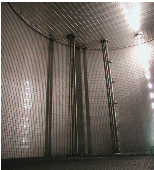
Figure 3. Inner view of a membrane full containment tank.
