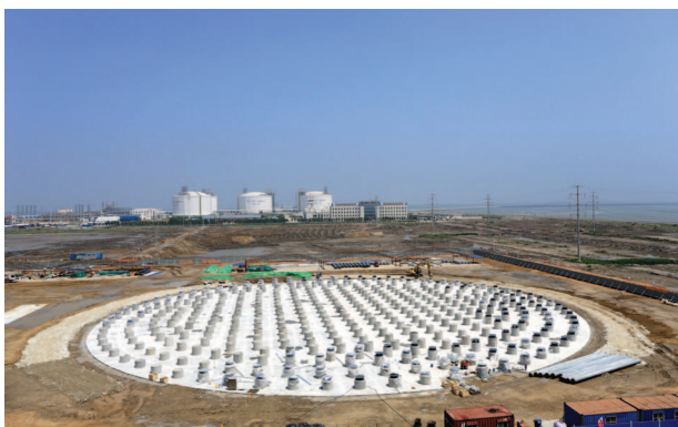
Figure 4. Completed fondation of the 220 000 m 3 membrane full containment tank in Tianjin, China.
