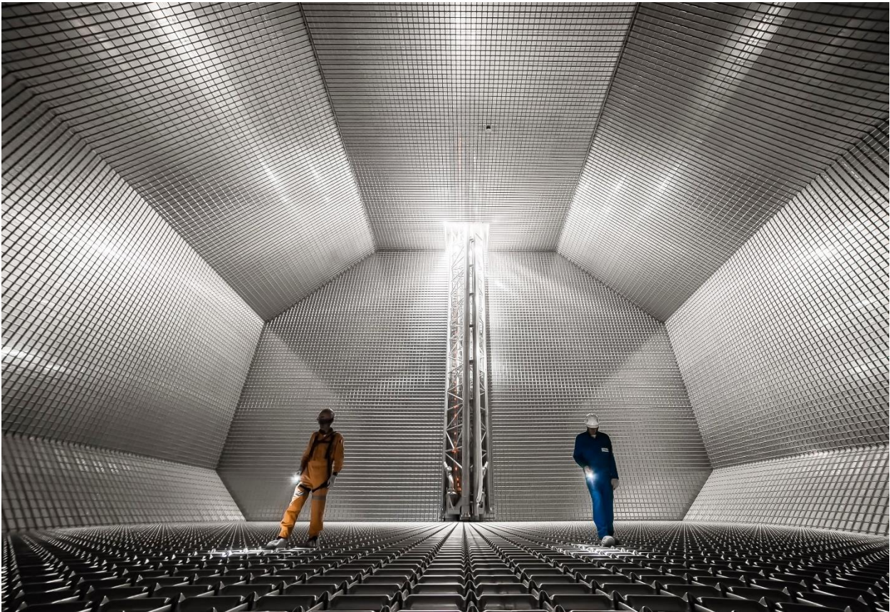
Caption: The inside of a GTT cryogenic membrane tank.
