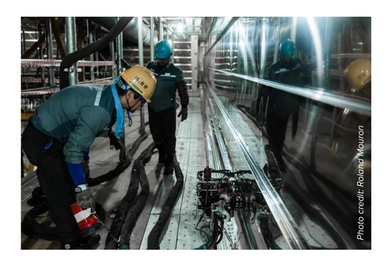
Workers use welding technology developed in-house at GTT to produce the company's NO96 LNG tanks.
