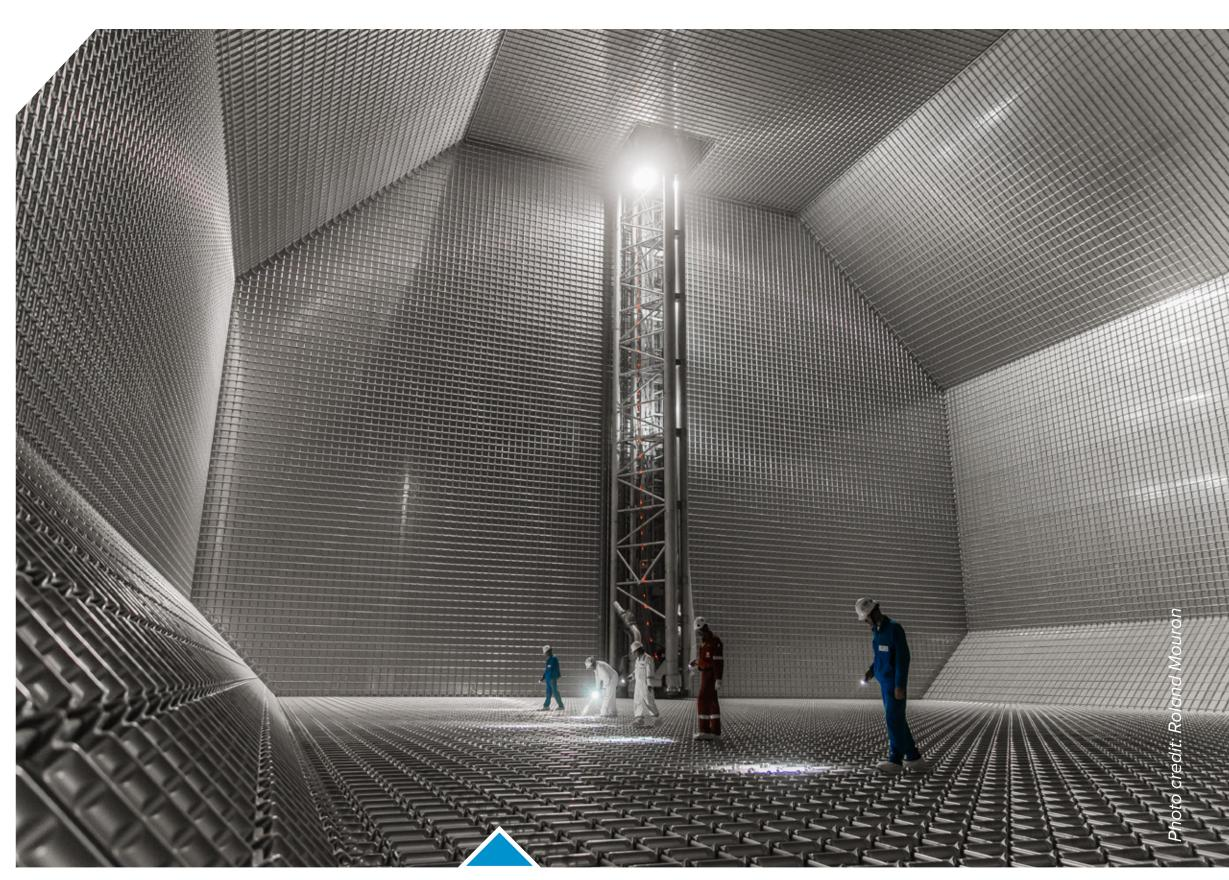
The inside of a GTT Mark III LNG tank where liquid natural gas will be kept at cryogenic temperatures.
